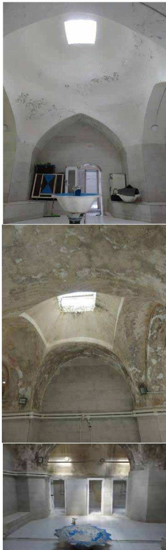
Fig. 9. Interior view of the Liqvan historical bathhouse. Source: Fereshteh Pashaei Kamali, 2022.
