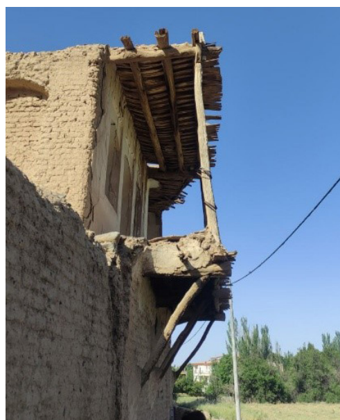
Fig. 6. The alley, an extension of life in the city. The Iwan of the house with a projection in the passage space indicates the extension of life in the house in the alley space. Photo: Alireza Afzali, 2025.
