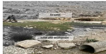
Fig. 4. The position of outlet before and after the development of the debouchure of the aqueduct and spring in Payastan village. Photo: Zeynab Rezaei, 2023.
