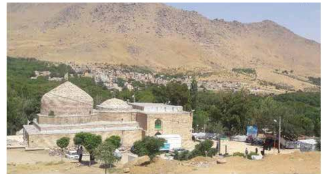
Fig. 4 the picture is related to 1996, the repair and renovation of the building, Photo: Reihaneh Khorramrouei, 2017.
